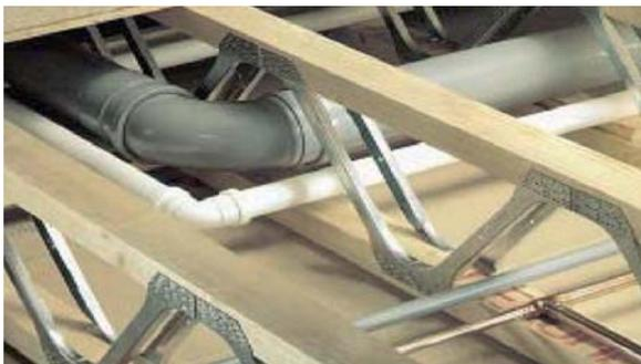
Open web joists easily accommodate services unlike solid joists.
